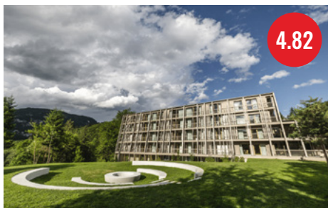
HOTEL BOHINJ BOHINJ, SLOVENIA
